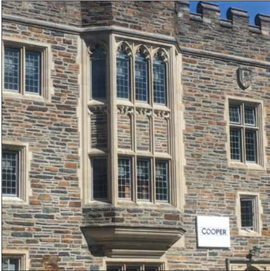
Residence Hall, Traditional
