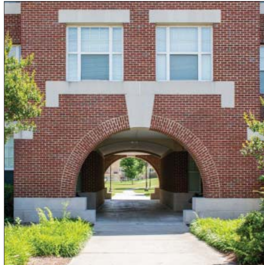
Arched passageway, Transitional
