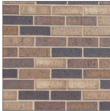
K4 Residence Hall - 2011
