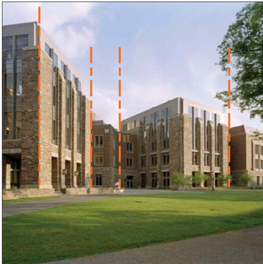
Large footprint broken into smaller parts, Fitzpatrick Center CIEMAS
