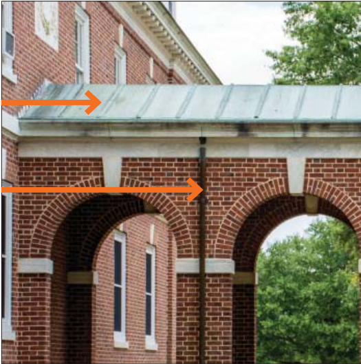
Copper roof & downspout, Traditional
