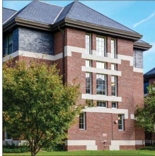
Pre-cast concrete, Transitional
