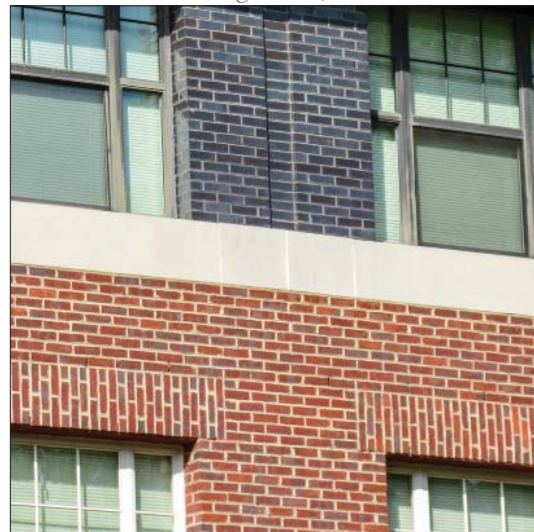
Pre-cast concrete string course detail, Transitional
