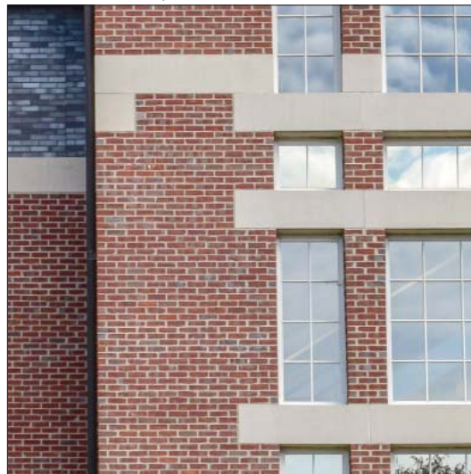
Pre-cast concrete detail, Transitional
