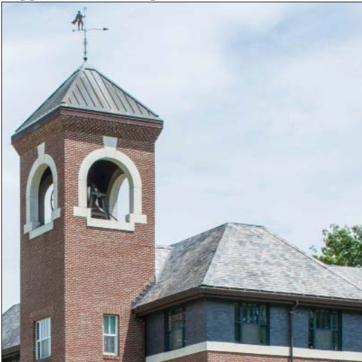
Slate & metal roof, Transitional
