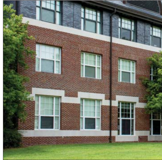
Pre-cast concrete string course, Transitional
