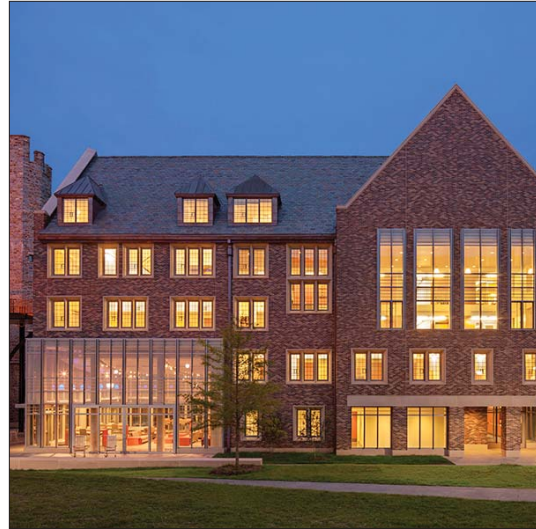
K4 Residence Hall
