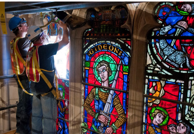
While the Chapel was closed, 7 windows were removed and restored and the mortar joints in the tracery were also repaired.
