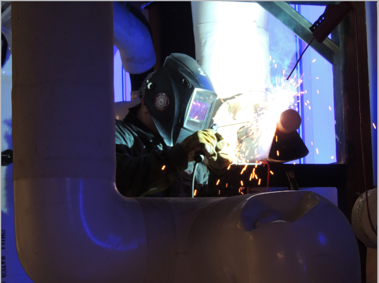
Steamfitter Ron Murphy works during a steam shut down in Cameron Indoor Stadium to replace the steam and condensate lines.
