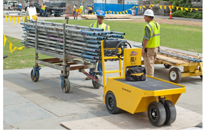
Scaffolding had to be built to create a work platform at the ceiling. The Chapel has no loading dock; everything came and went through the front doors.
