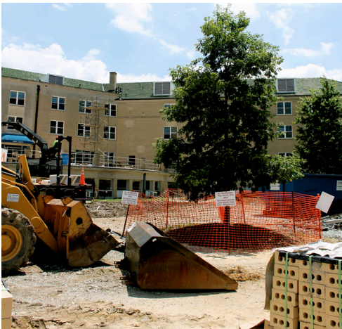
Tree roots grow like a dinner plate; shallow and close to the soil
