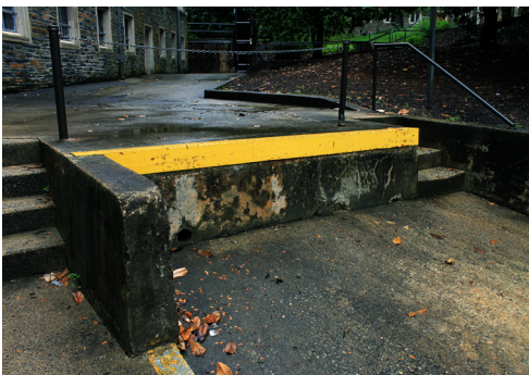
LOADING AREA Found on Allen Building
